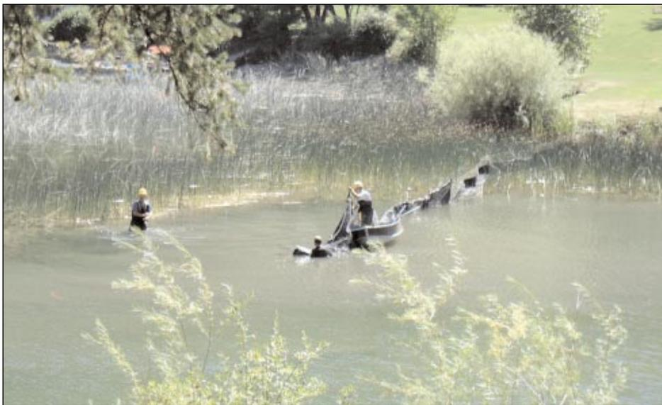
*The cofferdam site had to be completely isolated with silt fencing prior to dumping earth.*
